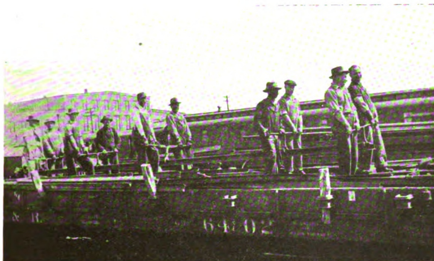
BEFORE. Old method of handling and sorting scrap rail.
