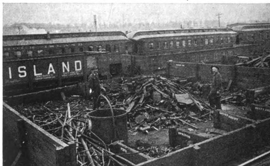
Sorting bin, Silvis scrap dock, showing how mixed scrap is received from the road. This is handled piece by piece, into the various classifications under which it is sold and the usable is accumulated and then taken by the crane to the reclamation shop.
