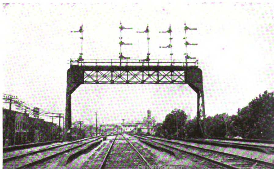
Westbound interlocking home signal, Joliet Union Terminal. UNIVERSITY OF ILLINOIS AT URBANA-CHAMPAIGN
