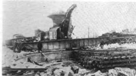
The steam wrecker was recently put into use to change out the turntable at Mantoy, Iowa, where improvements are being made.
