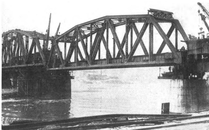
One of the greatest engineering feats in the history of bridge building was recently performed when the 435-foot span of the new Thirty-third Street bridge of the Baltimore & Ohio Railroad, across the Allegheny River, was rolled into position above the main channel in eight minutes. Two of the old spans were thus rolled up-stream in addition to the new span which weighs 3,000 tons. (Underwood & Underwood Photo.)
