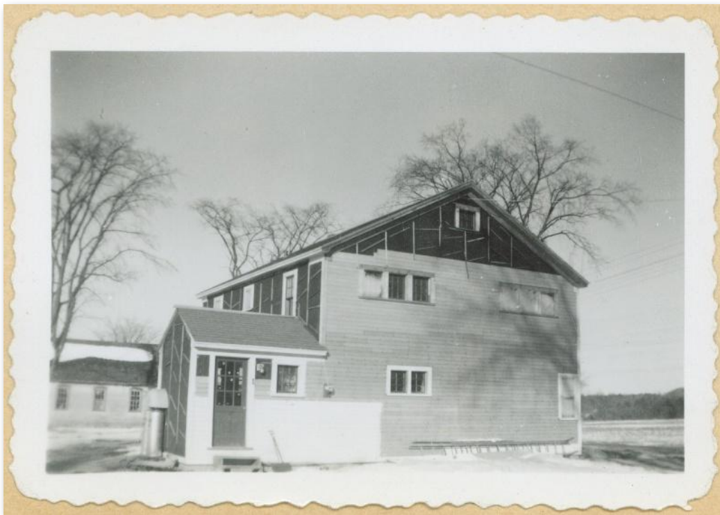
Figure 20 "South side with laundry. Clapboarding completed November 1950 after being in for a year."
