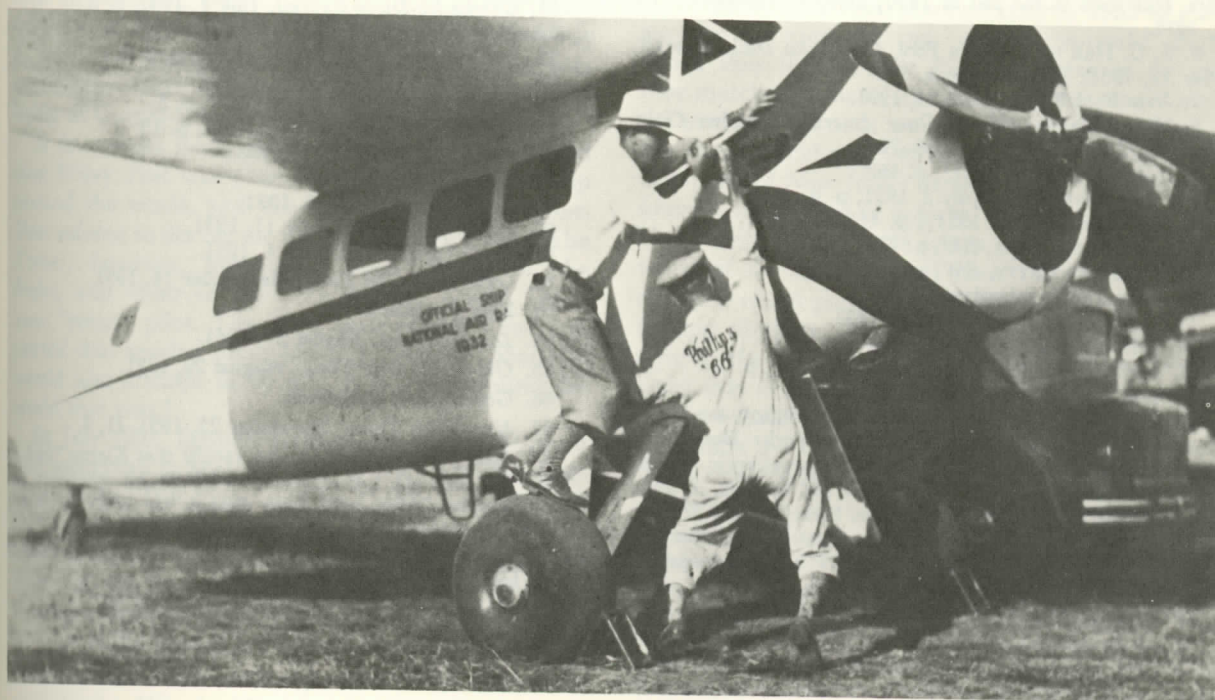
FIGURE 42.—Billy Parker's Lockheed Vega is started by hand-cranking the inertial starter at the National Air Races, 1932. The mechanic on the right is Fidel "Pancho" Vela, who maintained Parker's plane. (Courtesy Phillips Petroleum.)
