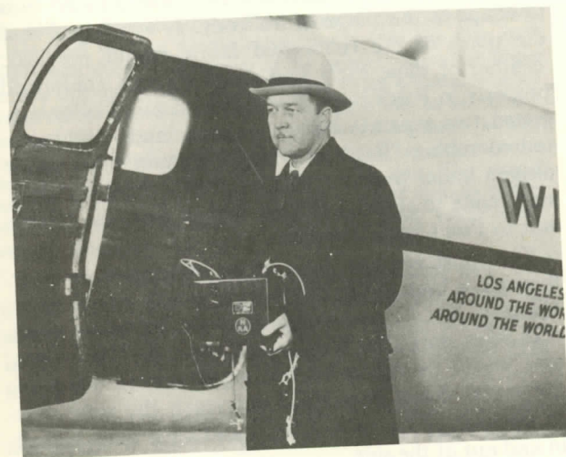
FIGURE 87.—A. M. Alcorn, Civil Aeronautics Administration inspector, prepares to install one of two sealed barographs in the fuselage of the Winnie Mae in December 1934, at Bartlesville, Oklahoma. These barographs were used in official record attempts in accordance with National Aeronautic Association procedures (note NAA initials on container). Shock cords for mounting are attached to the top of the barograph. (Courtesy Phillips Petroleum.)
