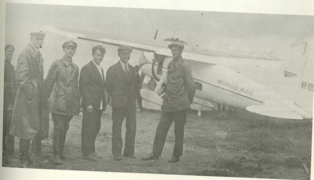
FIGURE 59.—The Winnie Mae is shown at Novosibirsk receiving the final servicing touches in 1933. One Russian is standing on the extendable steps on the left side of the cockpit, cleaning the windshield. Just below the fuselage window is an empty can of oil and the sense-antenna post may be seen on top of the fin, with the antenna running to the center of the fuselage at the trailing edge of the wing. Post landed in Novosibirsk at 6:27 a.m., and slept in the terminal building for two hours while the airplane was serviced. He took off at 8:55 a.m., the stop taking only 2 hours, 28 minutes. The efficiency of the stop service was responsible for assisting Post in beating the 1931 around-the-world flight. (Courtesy Fay Gillis Wells.)
