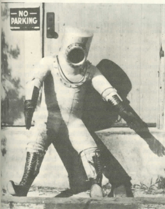
FIGURE 113.—A static pressure test is accomplished with Post's perfected flight-pressure suit after the Muroc forced landing, February 1935. Note the seat-belt marks above the thigh area and the outlet for the headset wire, just beneath the left, lower visor. (Courtesy Edwin O. Cooper.)
