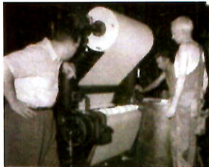
The original cloth laminator – Cloth was laminated to paper and the paper side was coated with an adhesive. Later, when complaints arose regarding the splitting of the paper, Charles Crowell invented the fiber-filled process which pre-split the paper, and then calendered it to give it a smooth finish for gumming. [What year was the photo taken?]
