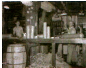
Workers slitting rolls of TUFFTAPE with the Kidder Slitter [What year was the photo taken?]
