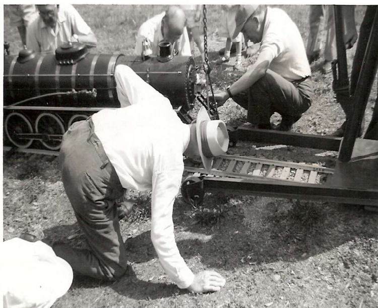
1961: AVRR volunteers re-rail engine 402 on the curve behind the Museum under the direction of Clarence Marshall (foreground).
