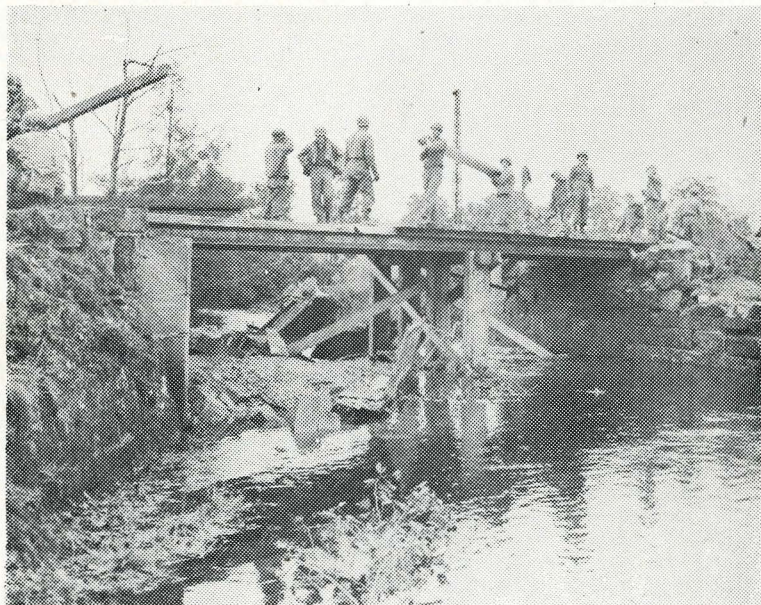
Engineers of the 120th Engineer Combat Battalion construct a trestle bridge outside Autrey, France near the end of September, 1944.
