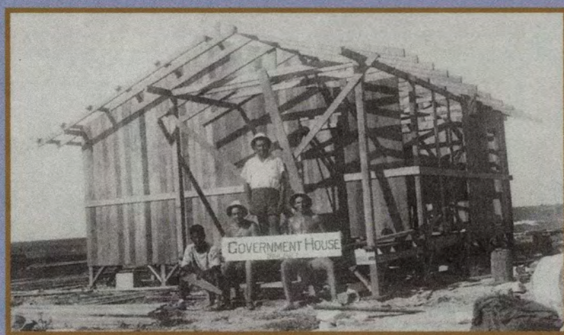
Harry T. Stewart, Territorial Architect for Hawaii, assisted in the construction of government houses on each of the islands, 1936. Photo courtesy of George Kahanu, Sr.
