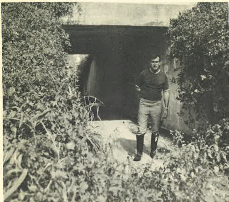
This tunnel runs under the viaduct. It was used by the small steam locomotive at the Long Key Fishing Camp.
