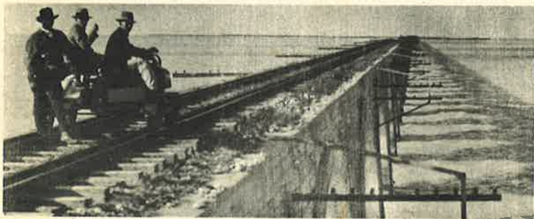
Hand car on the tracks of the Long Key Viaduct. Note double tracks, which is standard construction on bridges, to prevent wheels from derailing.
