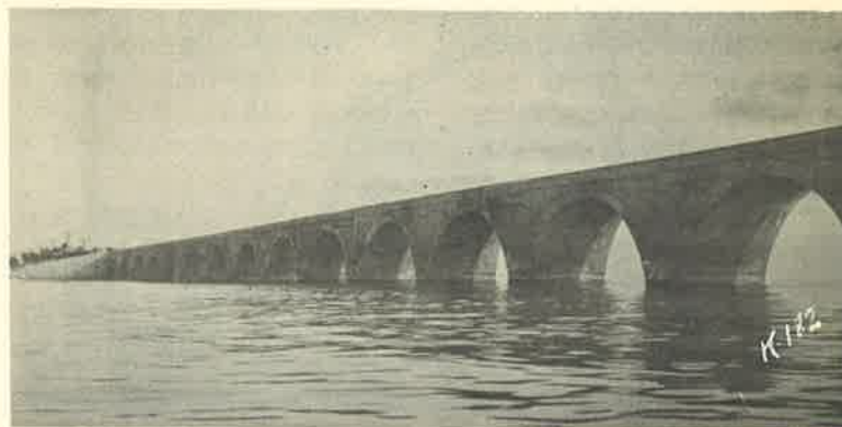
Long Key Viaduct, 1909, Belgium concrete was below the water line, above water, American cement.
