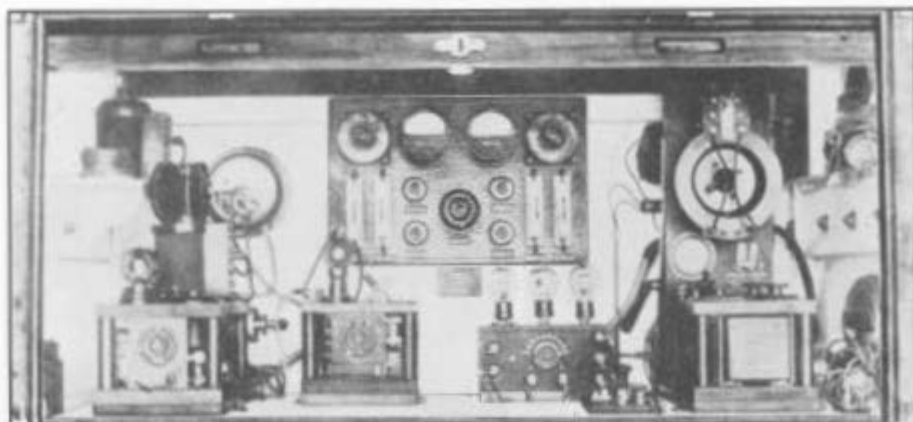
Fig. 40. Wireless Telegraph Set, 120 Watt, Mk I
