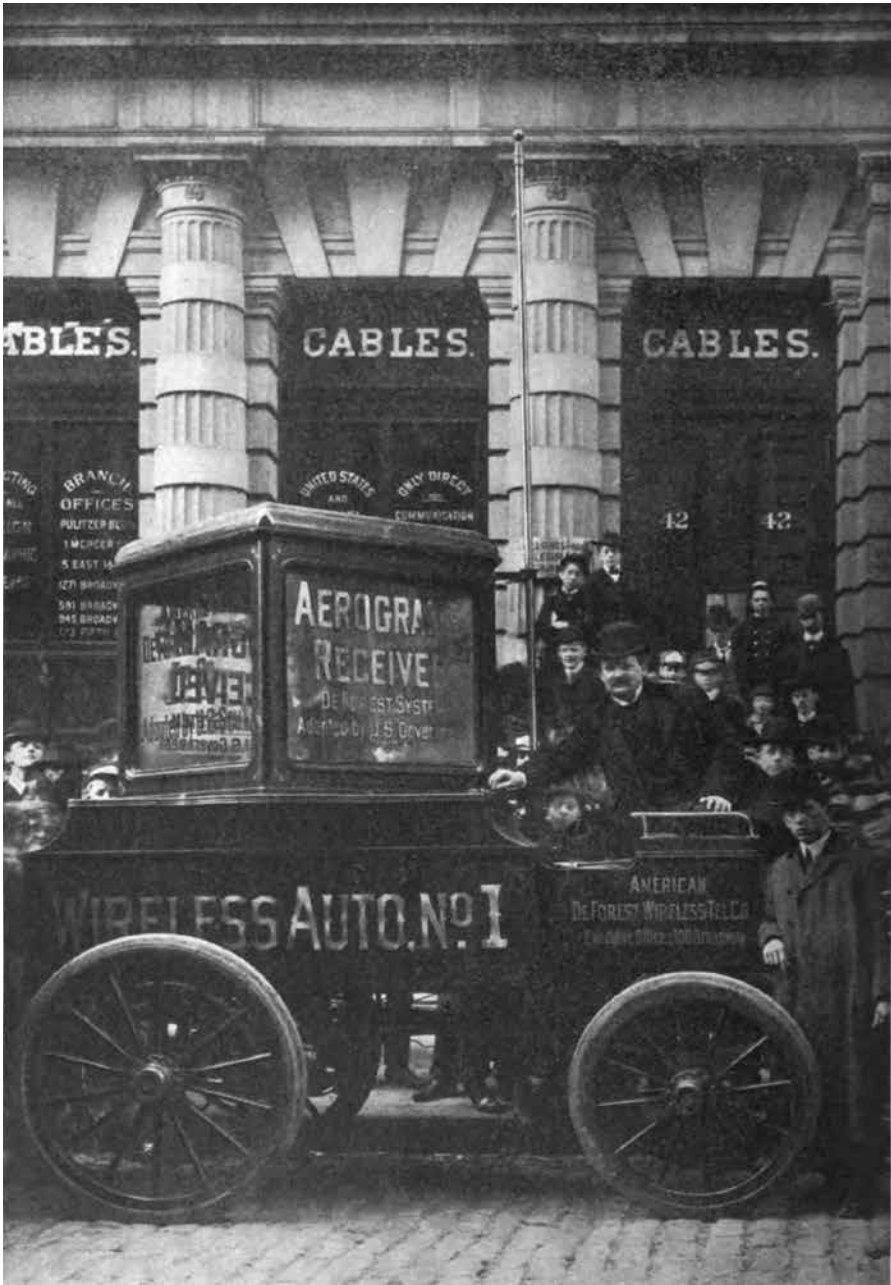
Fig. 22. This wireless automobile was one of two that were assembled by the De Forest Company as a publicity stunt to send stock reports from the curb to offices in the Wall Street area of New York, but in fact there was only the pretense of sending messages because the system did not work. ( Electrical Age , Mar. 1903, p. 178)
