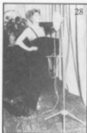
Fig. 28. Birdcage Stand with Modified Phonetron Speaker. Note "Distance" Rod on Stand.
