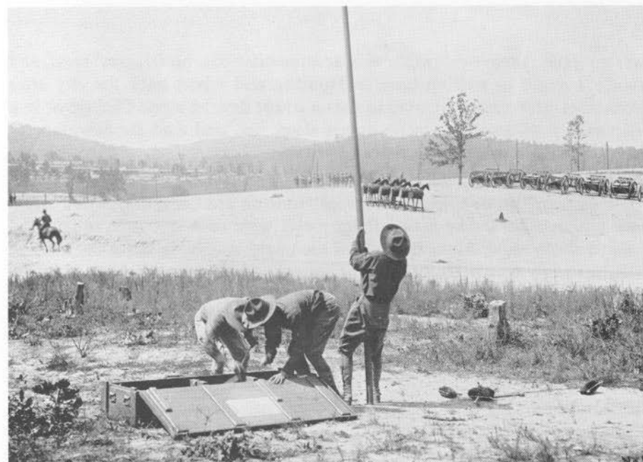
Fig. 5. Setting up a portable wireless installation. Note the row of "dummy" horses in the background.
