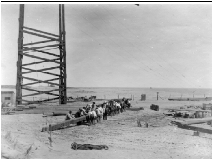
Figure 3. Erecting lattice towers at Glace Bay.
