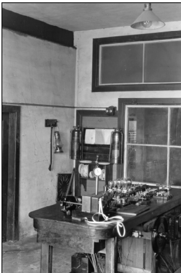
Figure 13. Condenser house, Glace Bay, May, 1912.
