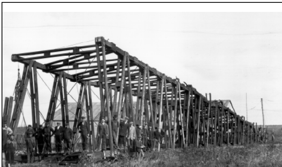
Figure 4. Glace Bay tower construction.
