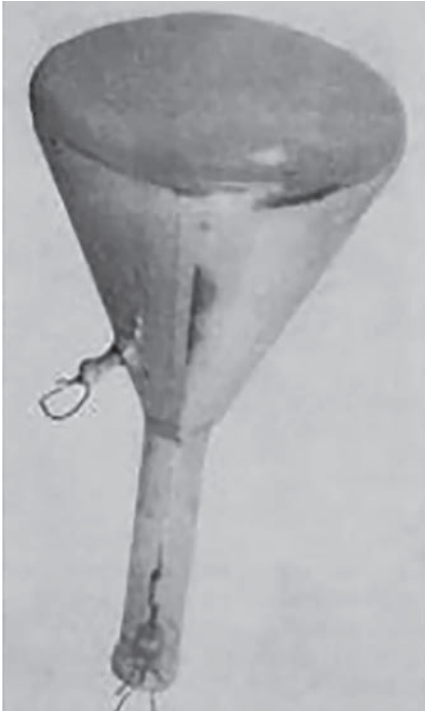
Fig. 20 Early DuMont Laboratories CRT used in experiments described in an article written by Allen Du Mont. ( Proceedings of the IRE , Dec. 1932, p. 1875)
