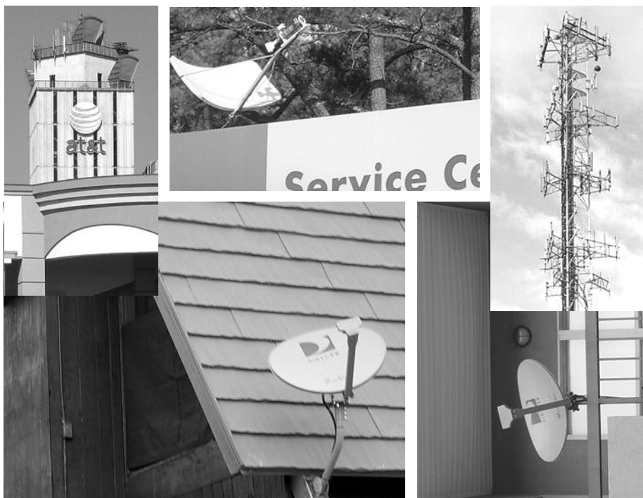
This collection of antennas for various services illustrates just how extensive the use of frequencies above 30 MHz has become. Clockwise from top: AT&T microwave antennas; satellite antenna used for data communications; cell phone antenna tower; satellite antennas used for television reception (two pictures).
