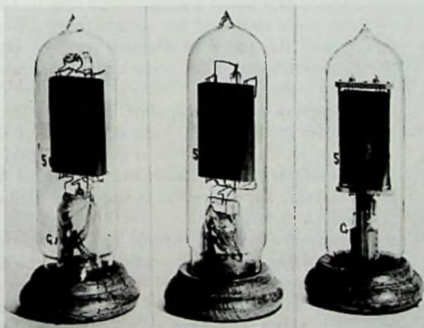
Fig. 14-11. Three experimental Type G tubes.
