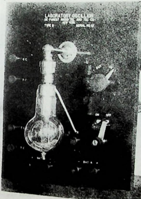
Fig. 7-3. The Type S Oscillation. (Reproduced from *Elect. Exper.*, Apr., 1917.)
