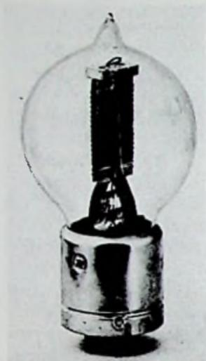
Fig. 14-21. The 217A vacuum tube.
