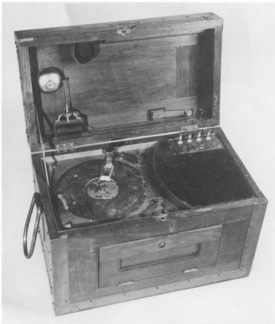
Fig. 5. The Beardslee A-B-C-type dial telegraph instrument of 1862-63. Most of these were destroyed.
