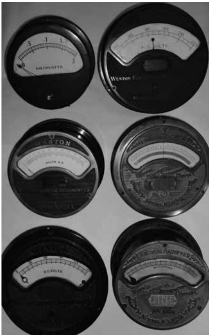
Fig. 15. Power station meters.
