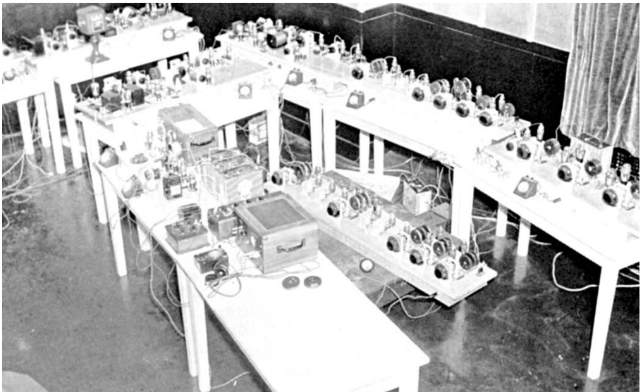
Armstrong's FM exciter equipment set-up in the Empire State Building in early 1934.
