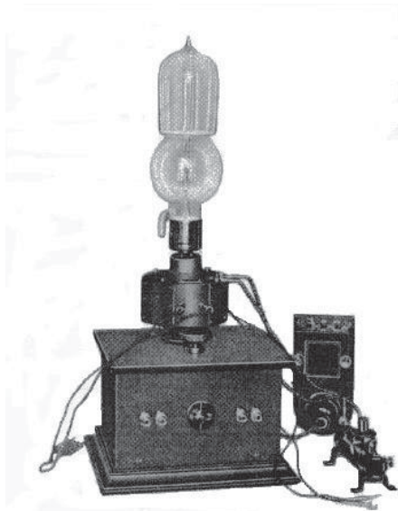
Fig. 10. Telefunken EV75 high-frequency amplifier, 1913. The EV72 audio amplifier had the same appearance, less the slide rheostat at the right and the circular assembly at the base of the tube. Source: Telefunken catalog .
