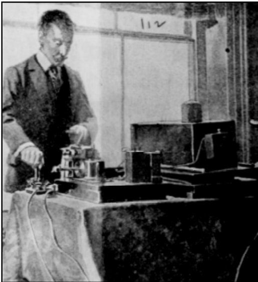
Figure 2. Sketch showing George Kemp transmitting with Marconi's first wireless key. Notice the method by which he grasps the handle.
