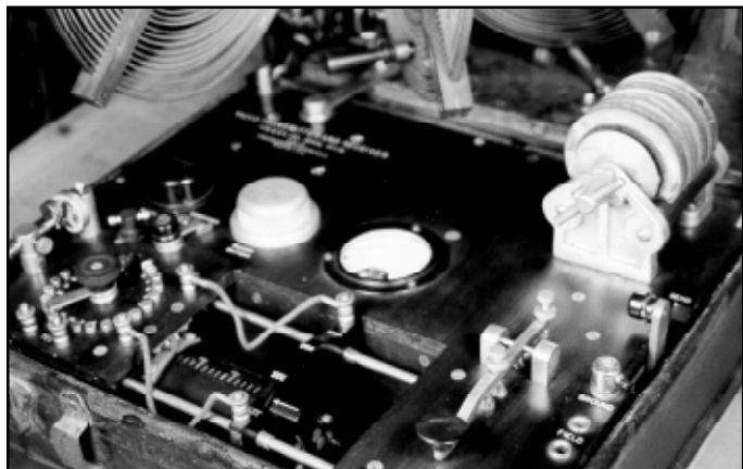
Figure 99. Close-up view of the key on the Wireless Specialty Apparatus Co. field set. It is similar to the Q-S-504.
