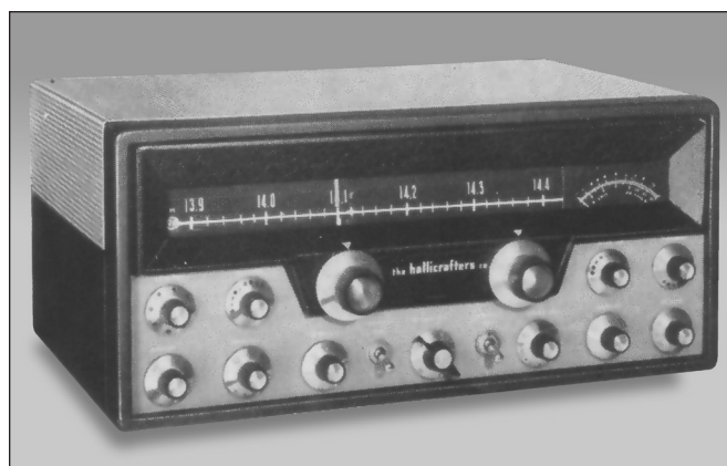
Hallicrafters' mostly solid-state FPM-200. Announced in the August 1957 issue of QST as "Coming from Hallicrafters laboratories," it was not a true transceiver. The unit shown was apparently a prototype as a very different looking finished product was announced almost two years later. QST, August 1957.
