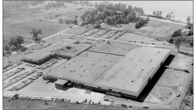
An additional 100,000 square feet of space was added to the north end of building in the mid 1960s. View to the southwest, with Lake Michigan visible at upper right.
