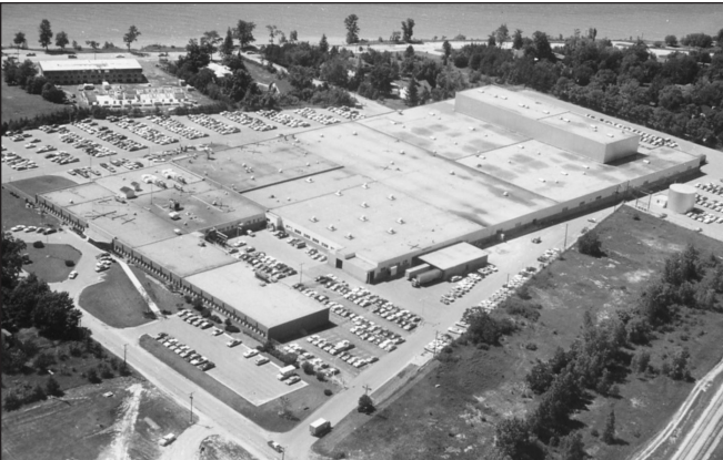
The stacker warehouse (upper right, with raised roof) was added in 1967. This brought the building to almost 500,000 square feet. View to the northwest.
