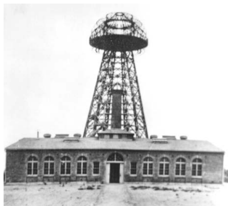
Figure 6. Tesla's unfinished Wardenclyffe station for his world system of wireless at Shoreham, Long Island, New York, circa 1903. The building in the foreground housed the power plant, laboratory, and workshops for the station. The tower and top structure in the background was about 187 feet (57 metres) high, and was never completed. The roughly hemispherical top was to have been covered with iron plates (the "elevated conducting body"), and the supporting structure presumably would have contained the "magnifying transmitter," and would have been covered by an outside wall.
