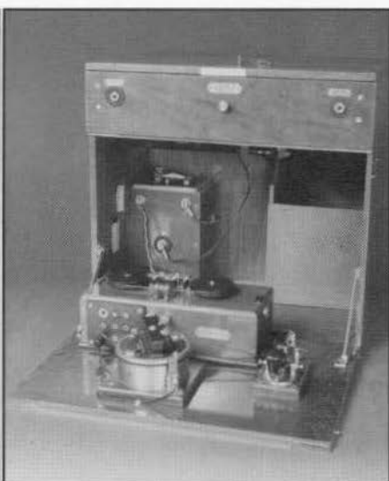
Figure 38. A prototype of Marconi's magnetic detector, used aboard the Italian Navy ship Carol Alberto in 1902. It was constructed in an ordinary cigar box. Source: Luigi Solari, Marconi, 1940
