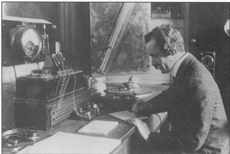
Figure 57. The receiving station at Clifden, Ireland. The magnetic detector is used with early type variable condensers and a multiple-tapped tuning coil.
