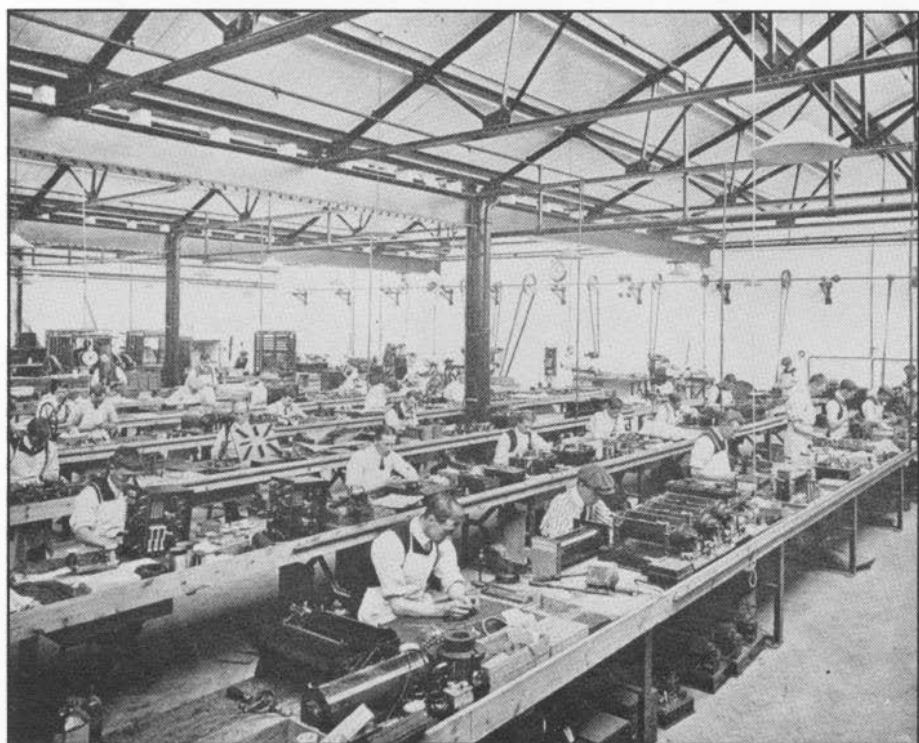
Figure 34. The mounting shop of the Chelmsford Factory, located on the 2nd floor, where the final assembly of transmitters and receivers took place.
