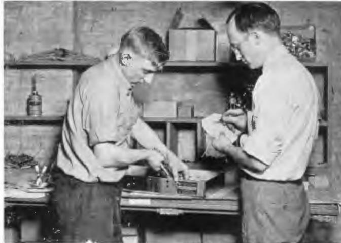
The first step in building every MASTERPIECE V is to rivet to its chassis the future owner's name plaque. From here on this receiver will be built to the exact specifications of its owner, accompanied by its own work ticket which goes through every step of assembly, test and adjustment with it. These specifications are on the work ticket in the hands of the engineer at the right, about to be tied to the chassis.
