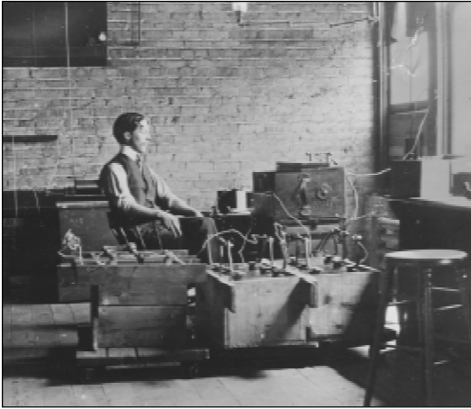
Figure 3. Wireless Station in Johnson Electric Service Co. factory
