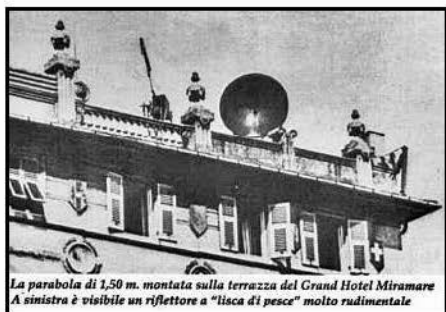
Caption translation: "The parabola of 1.5 meters mounted on the terrace of the Grand Hotel Miramar. On the left is a very rudimentary "herringbone" reflector."
