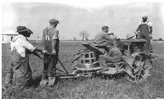
Figure 59. (Left) Ground radial installation for the vertical antenna.
