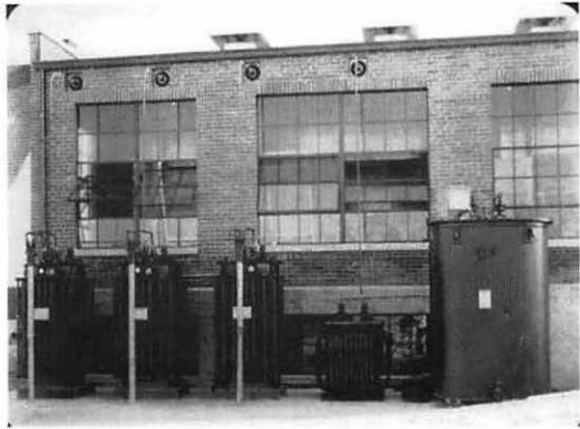
Figure 85. 500-kW transmitter plate supply single-phase transformers installed outdoors on the north side of the building. Also shown are the filter reactor and the modulation reactor.
