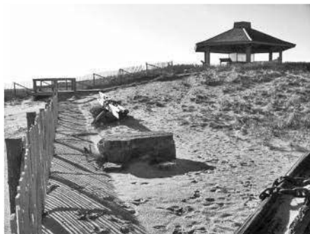
Pavilion before removal, tower remnants in foreground.
