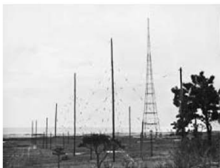
WCC—Receiving antennas at Chatham.
