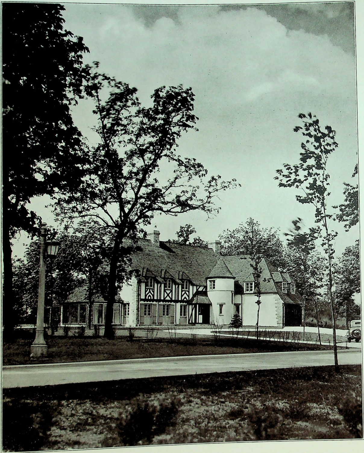
R ESIDENCE of Mr. and Mrs. Charles H. Starkweather, a charming example of Normandy Provincial architecture, in Verda Lane, of the "DEERPATH HILL" section, Lake Forest.
