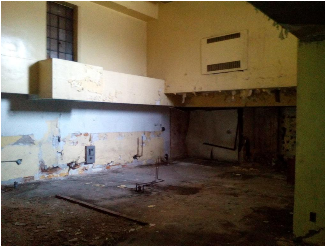
Former institutional Kitchen space
