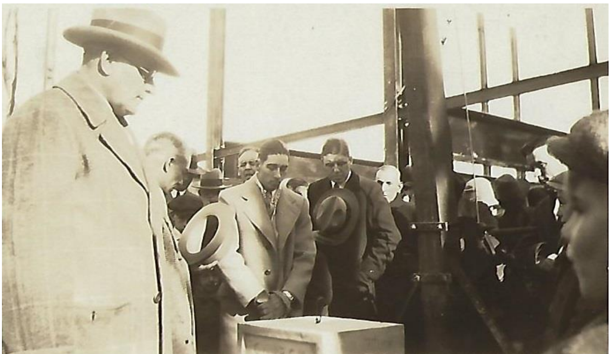
Laying the cornerstone, steel framework is seen in the background. Ca. 1928
