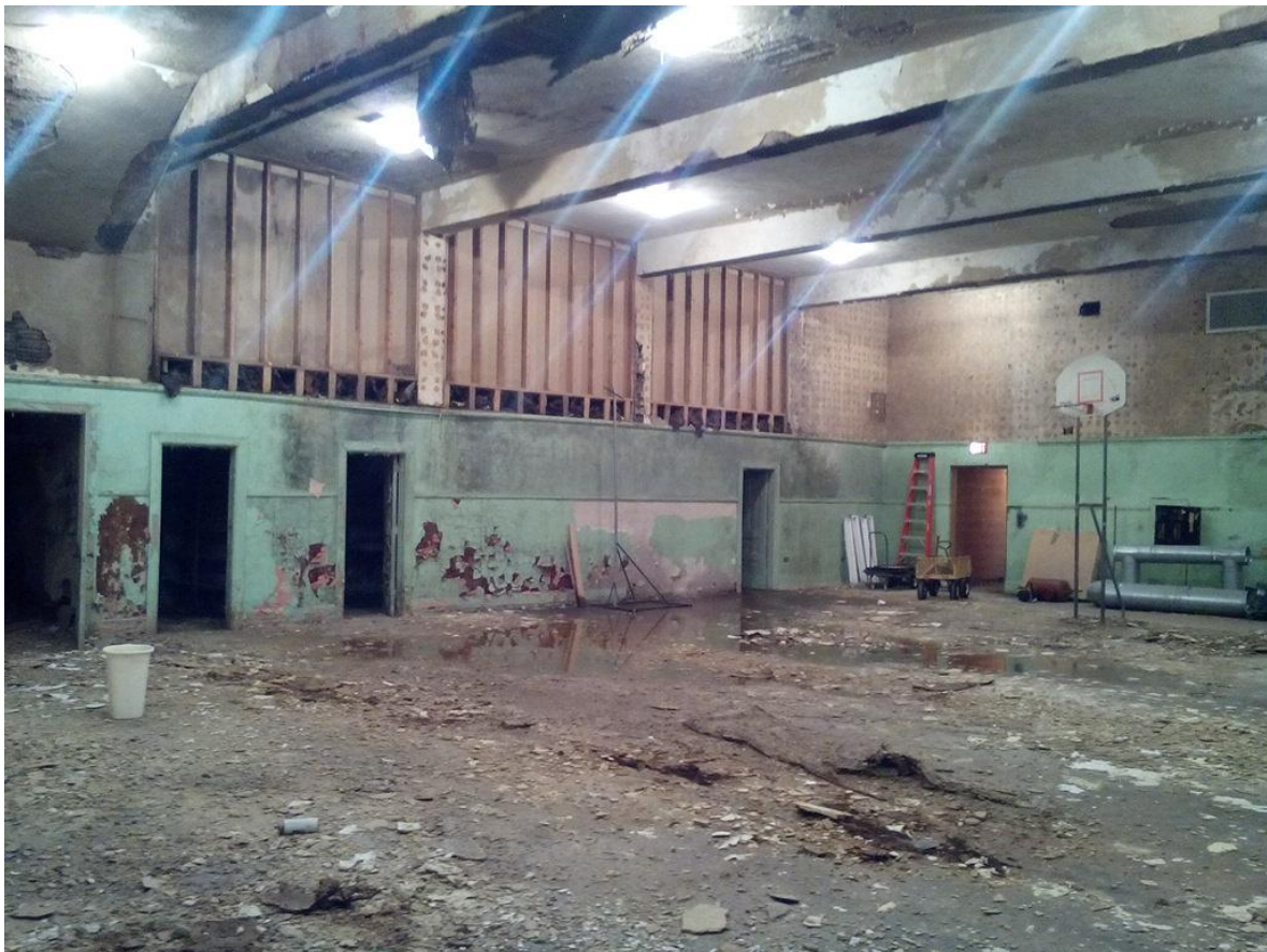
Gymnasium in the basement
