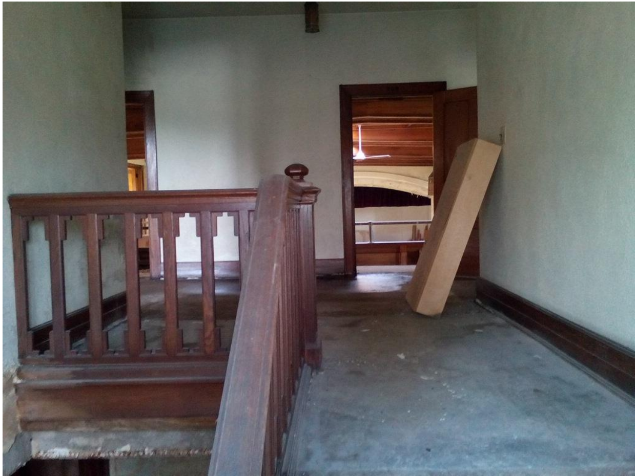
Second floor landing
