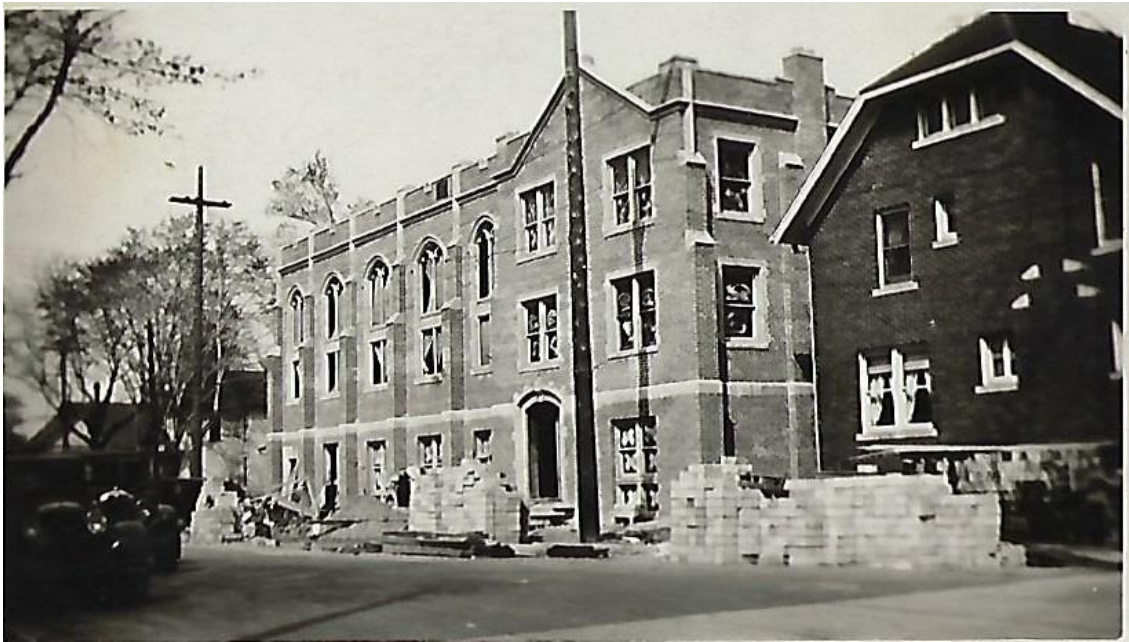
The building under construction. Ca. 1929. Former parsonage on the right.
