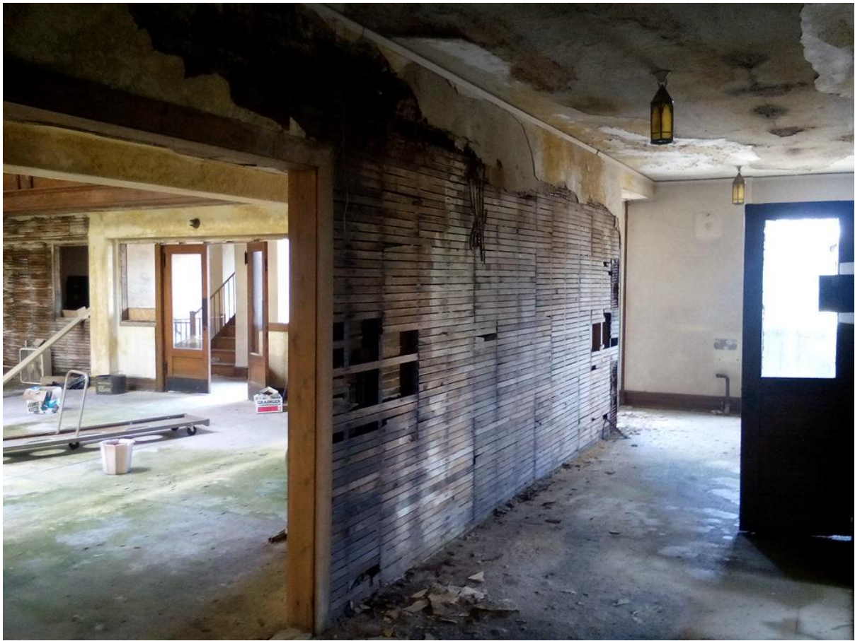
Condition of walls and ceilings throughout
