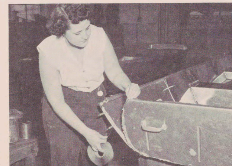
◀ Here, another worker applies sealing tape at the transom seam.
