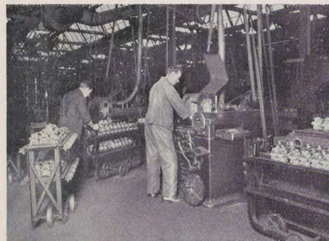
Experts making the shaft and crankcases for Britannia motors.
