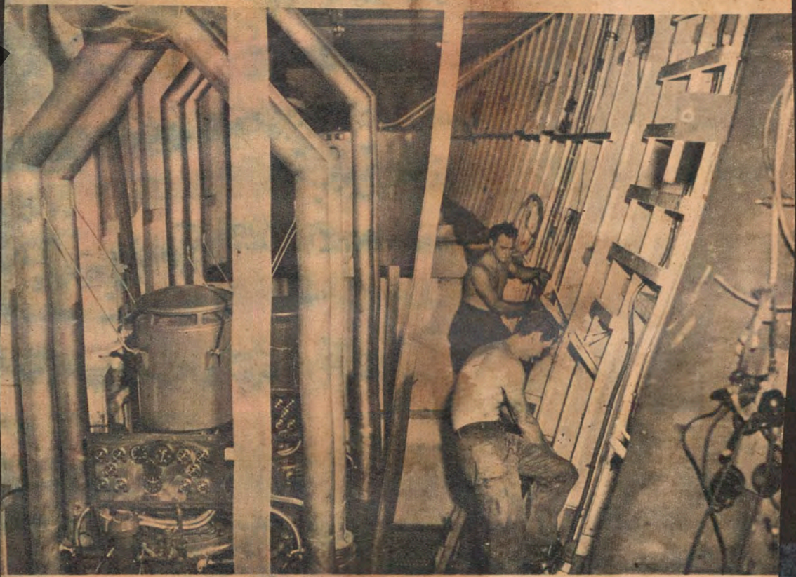
There's an engine room in each hull of the Venturi . This is the port room, looking forward. Powered by four 1200-horsepower pancake diesel engines, the ship has a cruising range of 3000 miles. Wood expects the vessel to be ready for public inspection in November.
