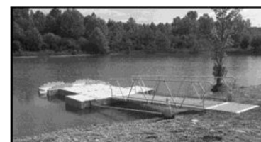
New Dock at Grand Valley
