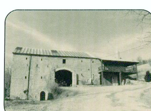
41 Kleinfelter Barn (1861) Magnificent three-story stone bank barn. Upper floors were used as a hay mow and for grain storage with livestock pens below. The porch addition is recent.
