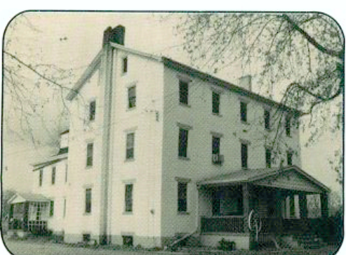
19 Office (1855) - ★ - Large three-story brick building served as Whitewater's central office. Visitors met with Shakers here to transact business, and could stay in rooms upstairs.
