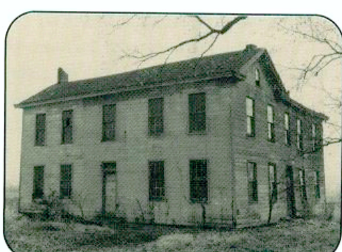
21 Broom Shop (1876) - ★ - Rare frame carpentry shop now in disrepair. Shaker products, such as brooms, furniture and seeds, were always of the highest quality and sold well in the marketplace.
