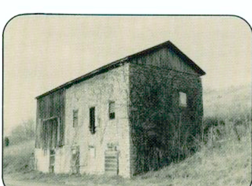
38 Horning Barn (c.1855) Very well preserved two-story stone bank barn with later frame addition. Features hand-hewn interior beams and a large arched stone doorway around back.
