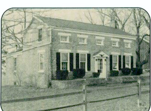
33 Hussel House (1862) Handsome stone house with massive lintels, small attic windows and a vaulted wine cellar. The farm, still family owned, also includes a small stone stable.
