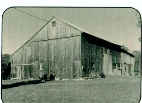
77 Sub-District School #4 (1879) Well preserved early barn features massive hand-hewn beams and wooden peg construction. Handsome frame farmhouse is nearby.
