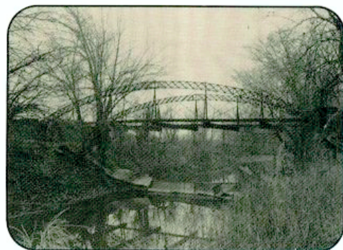
10 Zena King Bridge (c.1875) One of the few remaining bow truss bridges in the state. Zena King patented his innovative design in 1861. Built by the Massillon Bridge Company.
