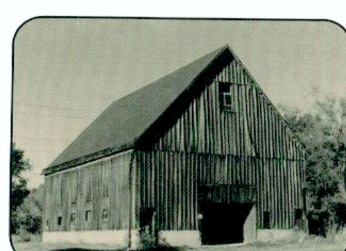
59 C. Rebel Barn (c.1885) Horse barn has stalls along both walls flanking a central corridor. The steep roof pitch and gable end doors are unusual features, note the board and batten siding.
