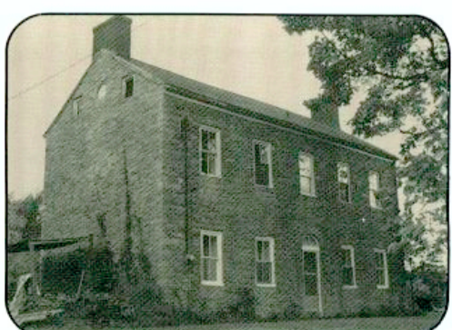
25 Werts House (1817) Very early Federal style stone farmhouse. Features include an arched fanlight, elaborate fireplace mantels, small gable end windows and hand-hewn floor beams.
