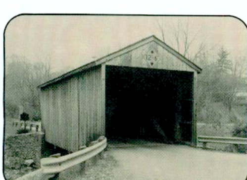
76 Jediah Hill Covered Bridge (1850) - ★ - Last covered bridge in the county and one of the few Queen Post truss designs in Ohio. Built by Jediah Hill, a farmer and saw mill operator.
