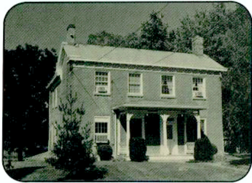
14 Wm. Sater House (1831) Fine brick house with Greek Revival details. The Saters owned an extensive farmland and were one of Crosby Township's most important pioneer families.
