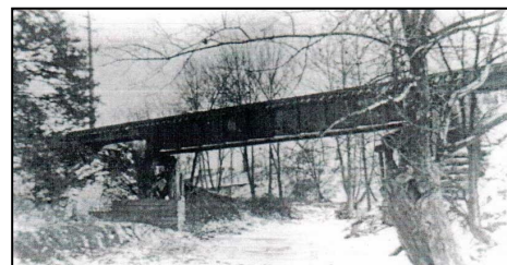
Swing Line bridge over Mill Run near Camp Stepping Stones
