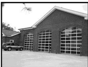
Emergency Vehicle Bay Doors Exiting to Drake Rd.
