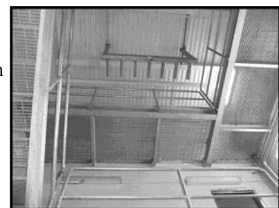
Interior View of Training Tower with Hose Drying Hooks
