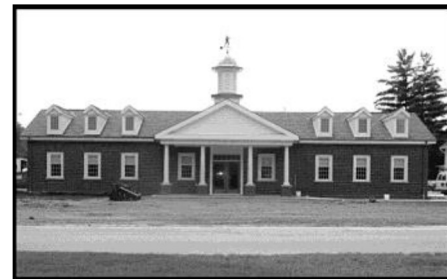
Firehouse Entrance on Shawnee Run Rd.
