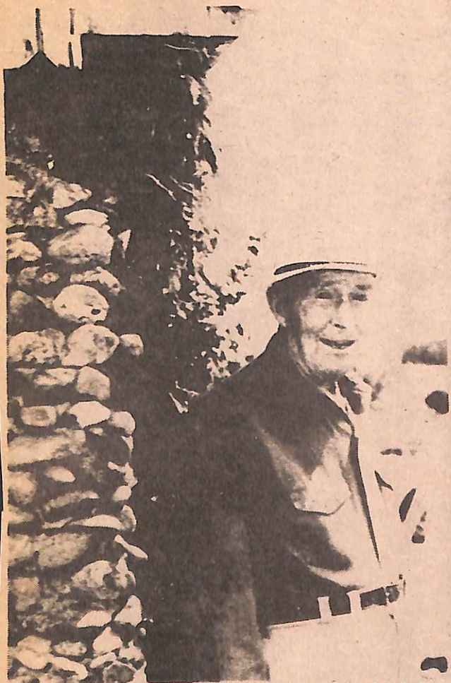
Percy Marion stands by the porch post he built from field rocks.
