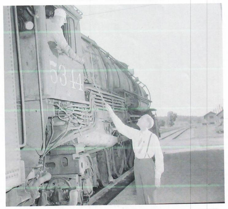
As trains passed by stations placed at regular intervals along the railroad, train orders received by telegraph operators could be handed up to passing trains through the use of message hoops. To take the message, the engineer caught the wide loop of string in his hand. The Telegrapher would then place an identical message in the hoop again for the conductor who usually rode in the caboose at the end of the train.
