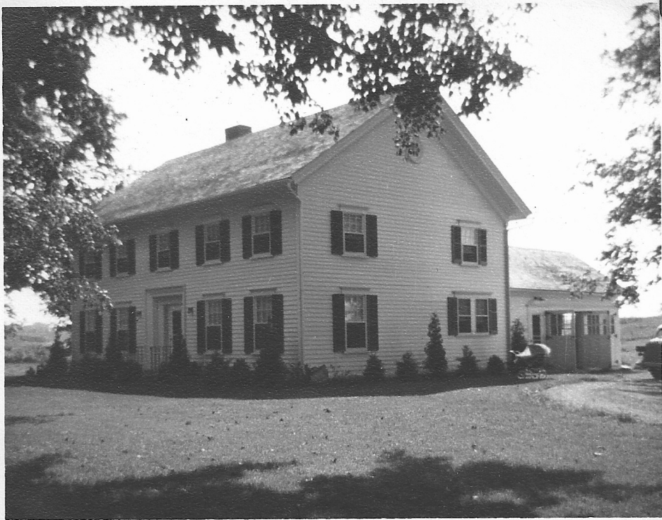
J. Schneider Elyanille farm remodeled Former Mellen & Moore
