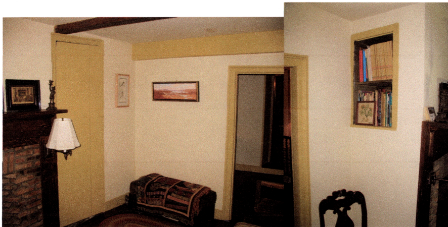
Cupboard is original: Very wide board, trim and remains of HL hinges Original trim around doorways. Low and wide doorway. Warming cupboard built into chimney.
