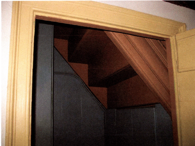
Bottom of early 18C enclosed stairs leading to upper storey. Note molding intended for decorative effect.
