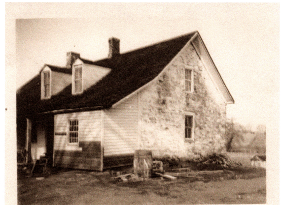
1940 North gable side. Note original and replaced clapboards. Eave overhangs.
