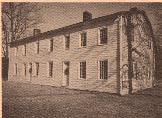
The west facade of the Inn was restored in 1984. The work included the reproduction of the 12 over 12 sash on the first floor level. This work was based on a surviving 18th century window on the east side of the building.
