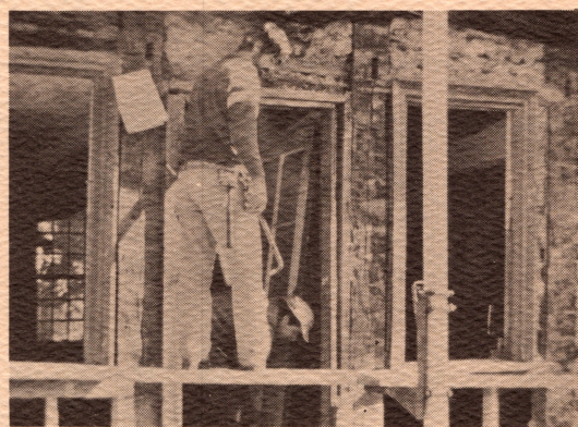
Carpenters from Craft Construction Company discovered mud and straw insulation dating from the 18th century when clapboards were removed from the north end of the building. The original clapboards were replaced after repairs were made.
