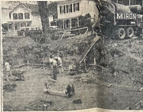
Concrete for footings is poured at the site of the new First National Bank of Red Hook building. The photo above, taken on May 11, 1959, was only a few weeks after excavation work had begun on April 16. The old Kelly Nursing home was purchased by the bank and torn down to make way for the new building. Standing near shore are from left to right, Harold Pollman, foreman for the Velletri Construction Co., James S. Griffin and B. Buffington.
