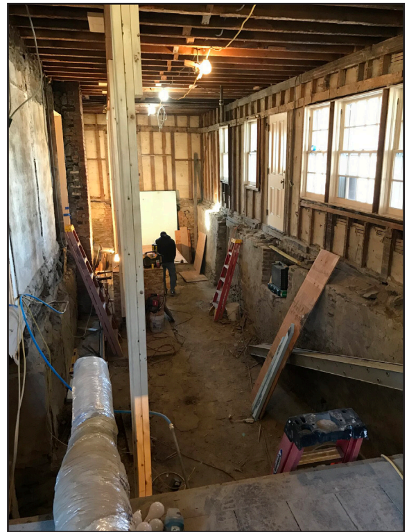
While the Martin Homestead's circa-1870 rear wing requires some new structure, perimeter framing is being reused.
