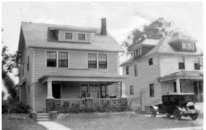
The sidewalk to the house now leads to the corner of a new front porch.
