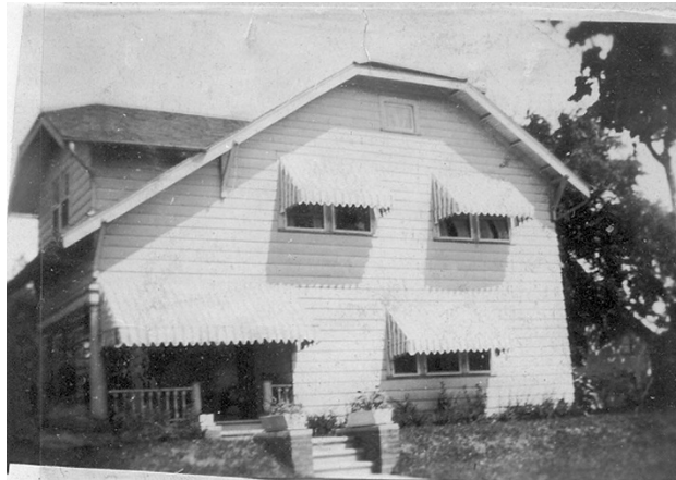
633 Allison Avenue before the tornado
