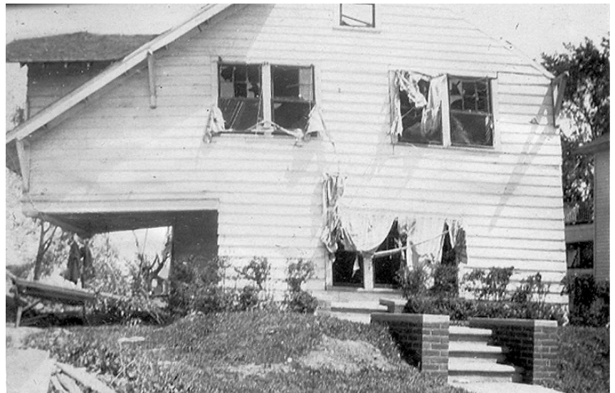
The house was torn from its foundation and moved north. Note the position of the porch to the walk and front steps.
