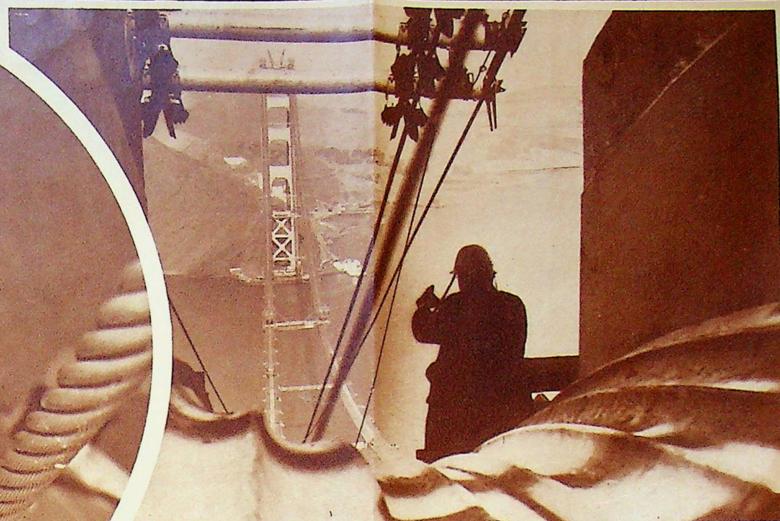
Looking over a 169-ton cable saddle toward the north tower.
